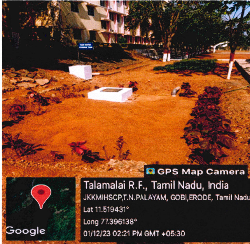
PHOTOS OF INSIDE VIEW RAIN WATER HARVESTING STRUCTURE
