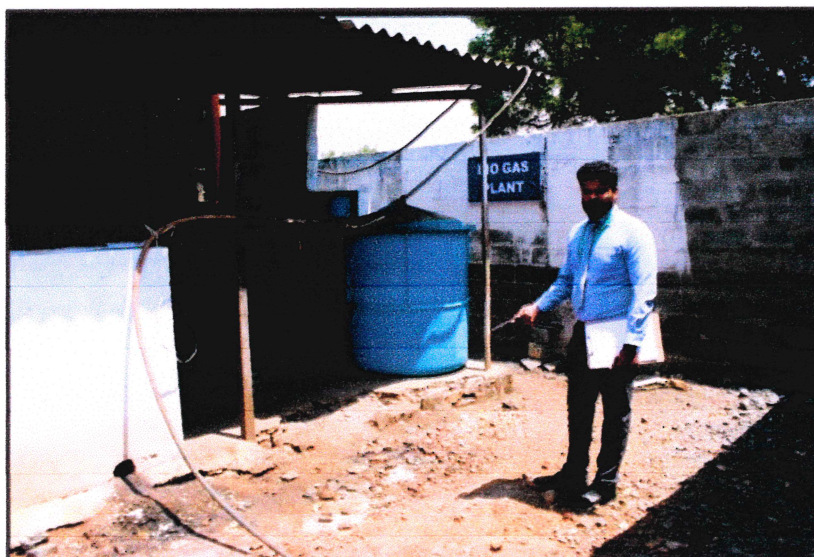
Biogas unit in the College Campus
